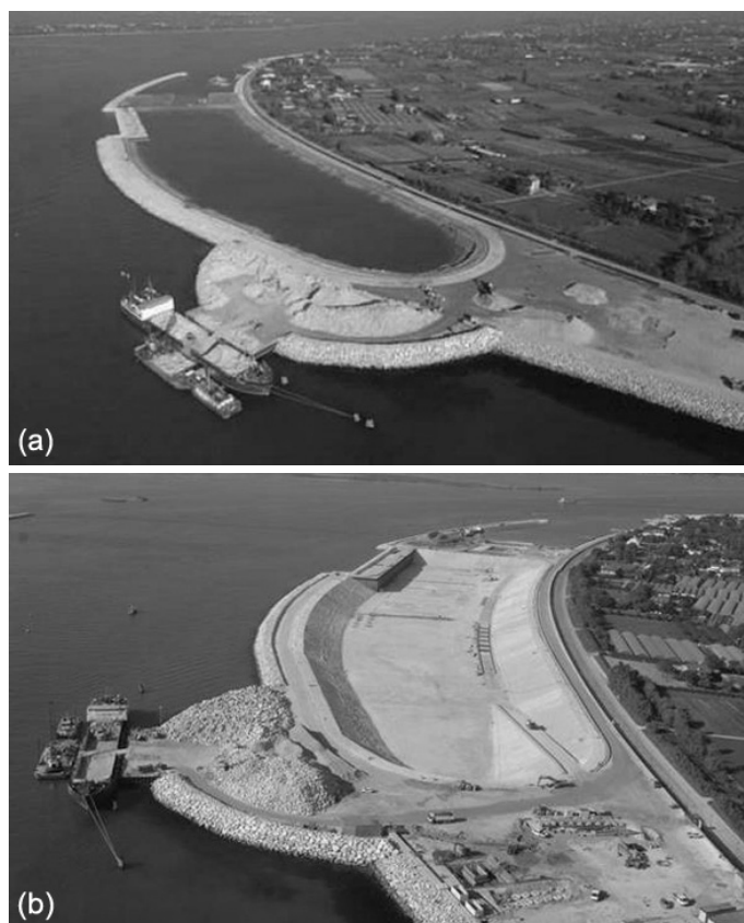
Figure 1. Harbour construction: (a) before and (b) after dewatering operations.
